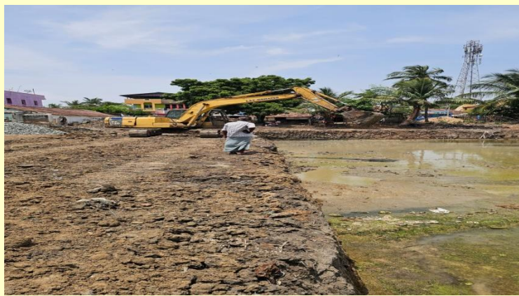
Levelling the area around the Teertham and creating an entrance pathway using a JCB
