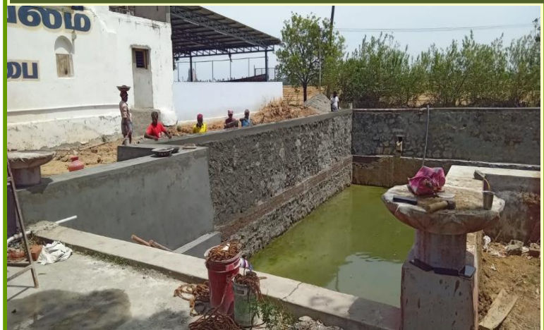
Final plastering work is on ....
