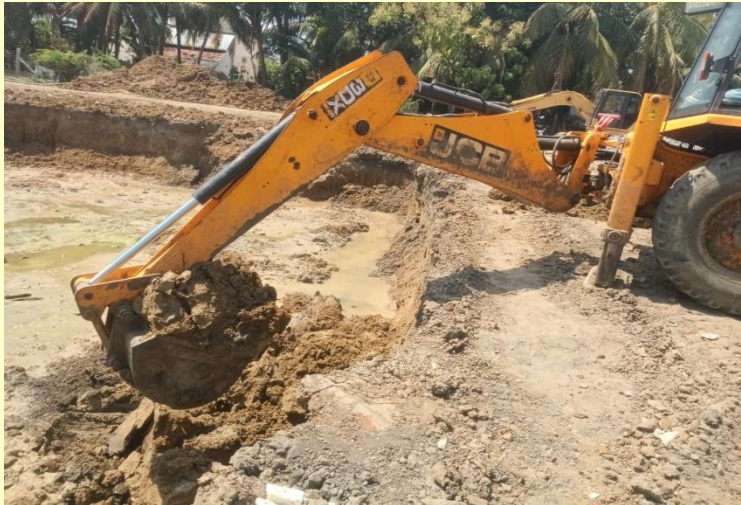
Excavation is going on by using a JCB
