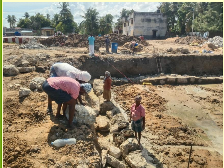
Foundation work is on ...
