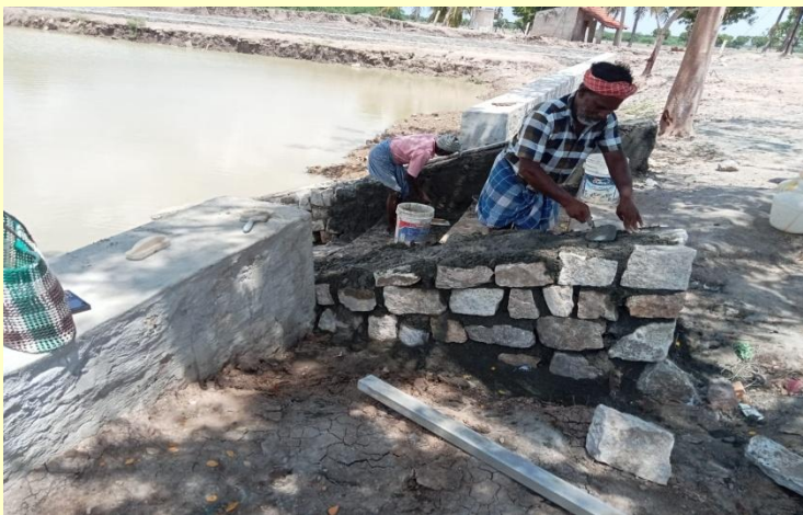
Retaining Wall Completed - Entrance step work underway
