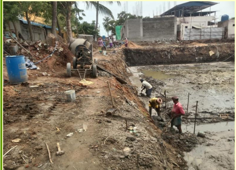
Taking the extra soil from the side bunding for shaping the Teertham
