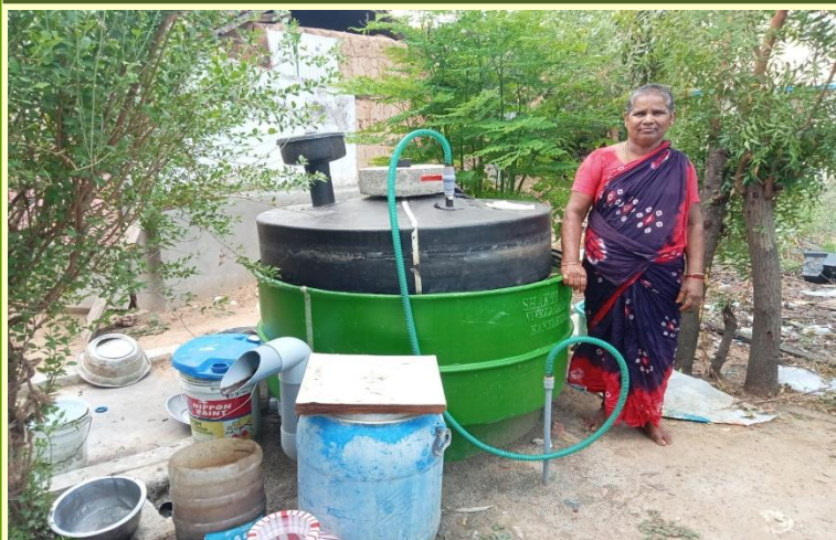
From Waste to Energy - Smt. Shanti's Green Initiative
