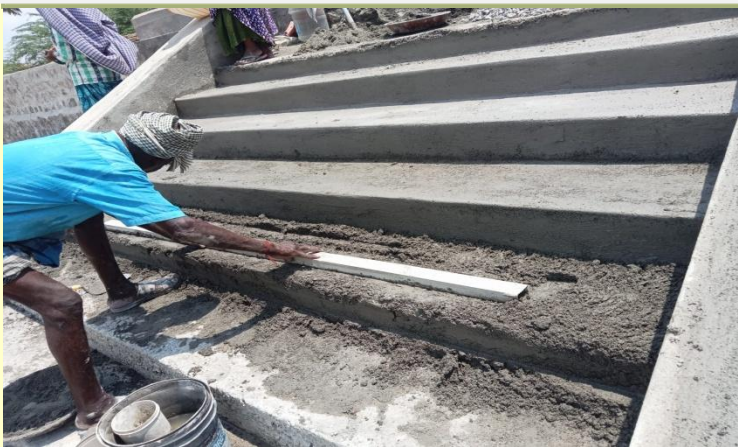
A Finishing Touch - Step Plastering Underway
