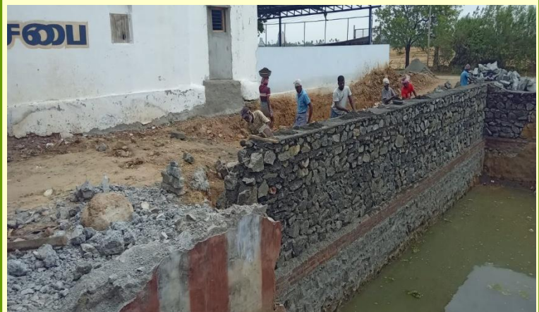
Construction of the stone retaining wall is underway to strengthen the water body's banks and ensure its long-term stability
