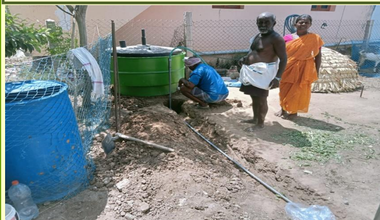
Pipeline installation work is underway to connect the biomethanation plant to the household kitchen - Shri.R.Gandhi
