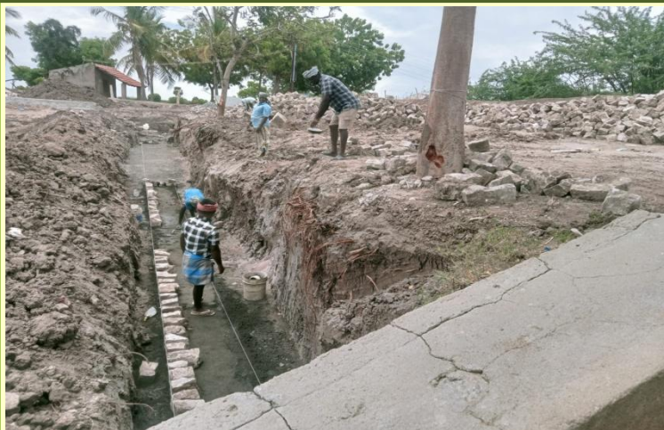
Foundation work is on ... for the wall construction
