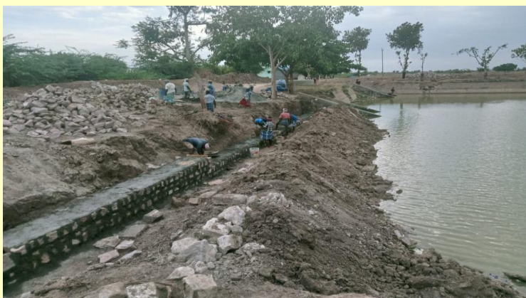
Slowly and gradually, the wall is taking shape
