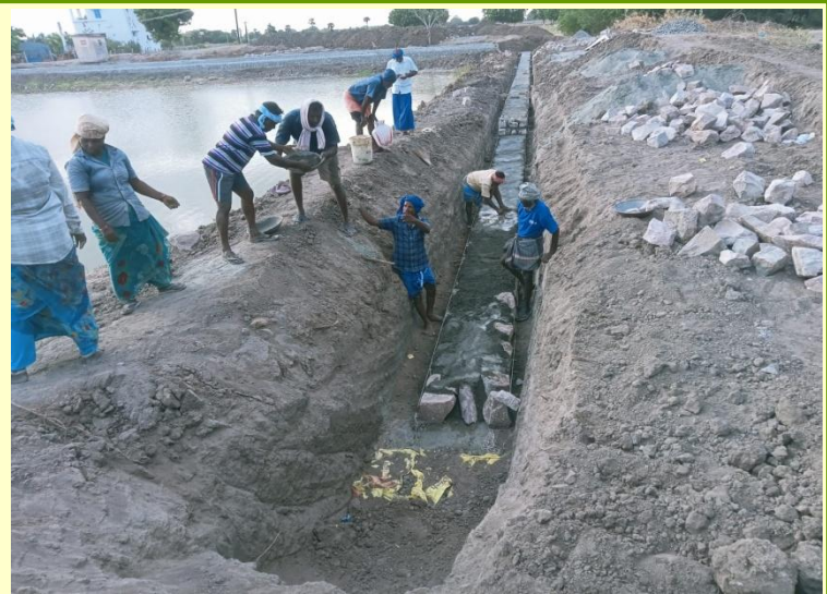
Foundation work is on for the wall construction
