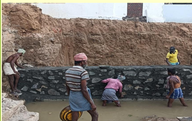
Slowly and gradually the wall is taking shape. Workers doing the work by standing in the water
