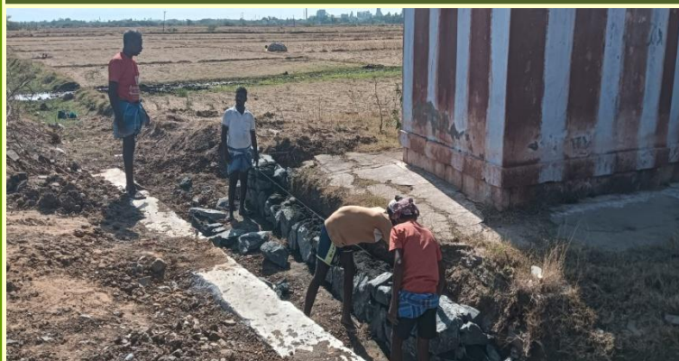
Solid foundation work is on for the broken wall construction
