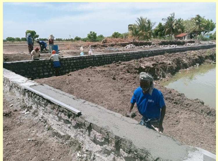
Slowly but steadily, the retaining wall is taking shape and has now reached the parapet level, marking a significant milestone in the restoration of the water body.
