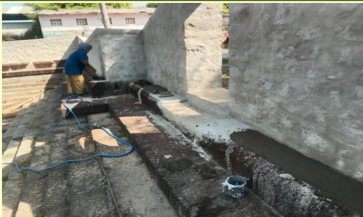
Washing the area before starting the white washing work
