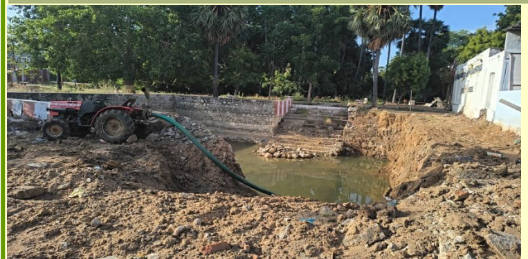
Pumping out the water before reconstruction
