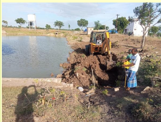
JCB-Assisted Site Grading and Excavation for Retaining Wall Construction
