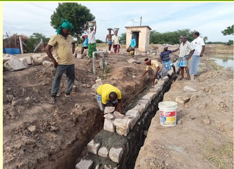
Construction of retaining wall with sound foundation is on ...
