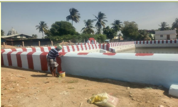
Workers giving traditional colours - white and Kavi to the renovated temple tank
