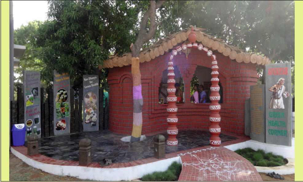
Rejected mangalore tile arch
