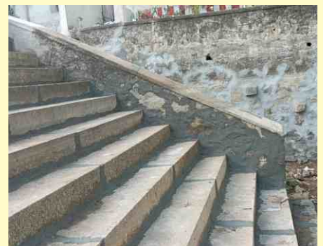
Strengthening and pointing of steps
