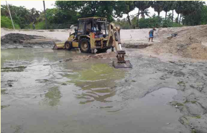
De - silting and Deepening the water body
