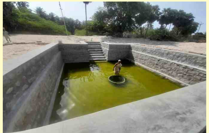
Construction of Inner pond and ring well
