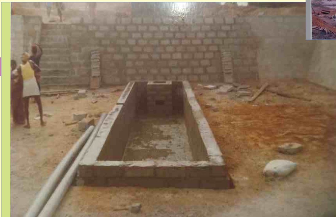
Digging of tube well and Horizontal sand filter
