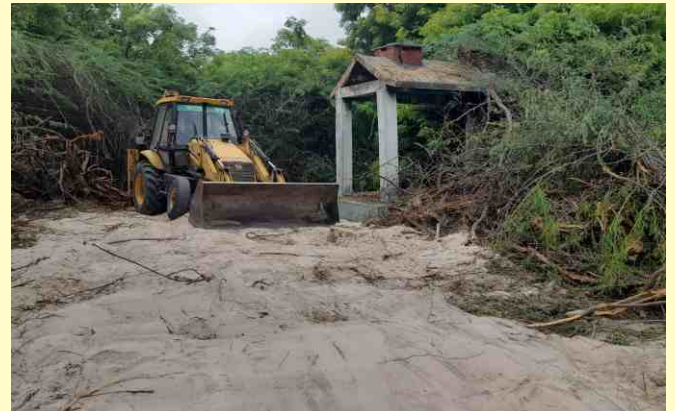
De - silting and Deepening the water body
