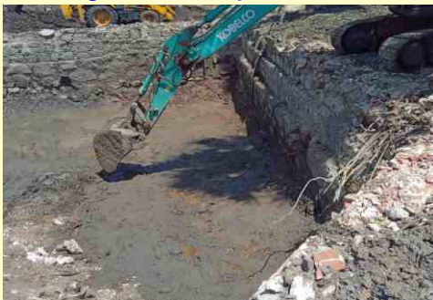
Desilting with the help of JCB & Tractor
