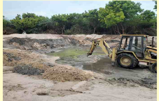
De - silting and Deepening the water body
