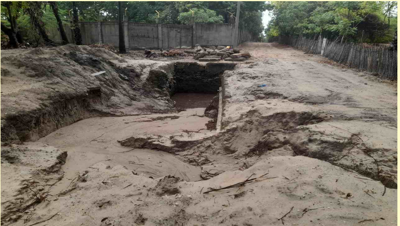
Traditional water body before renovation
