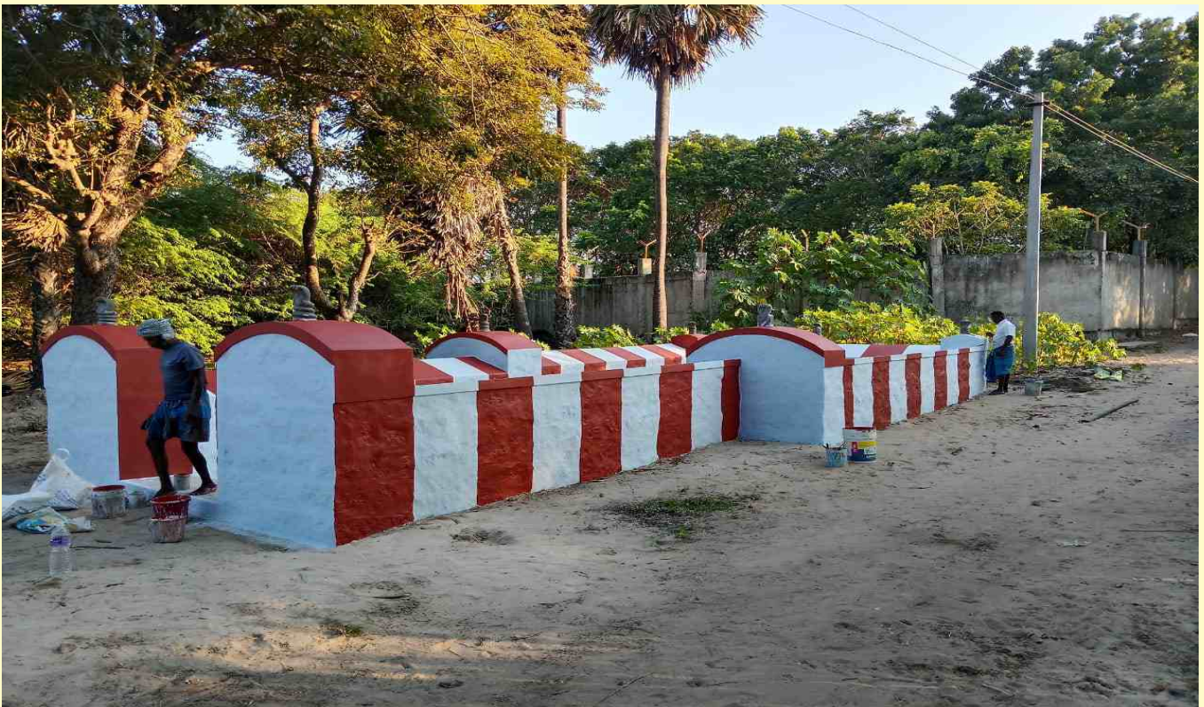
Teppakulam - After completion of the work
