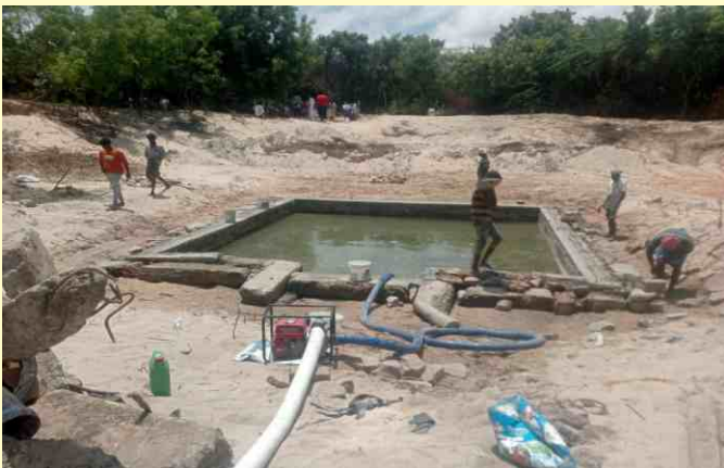
Construction of Inner pond and ring well
