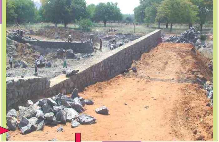
Excavation and construction of side walls
