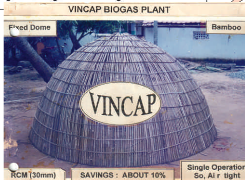
VINCAP model developed by VK-NARDEP uses locally available and cost-effective building technologies. This brings down the cost by 12-20 percent.
