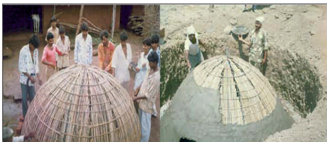
VINCAP model developed by VK-NARDEP uses locally available and cost-effective building technologies. This brings down the cost by 12-20 percent.
