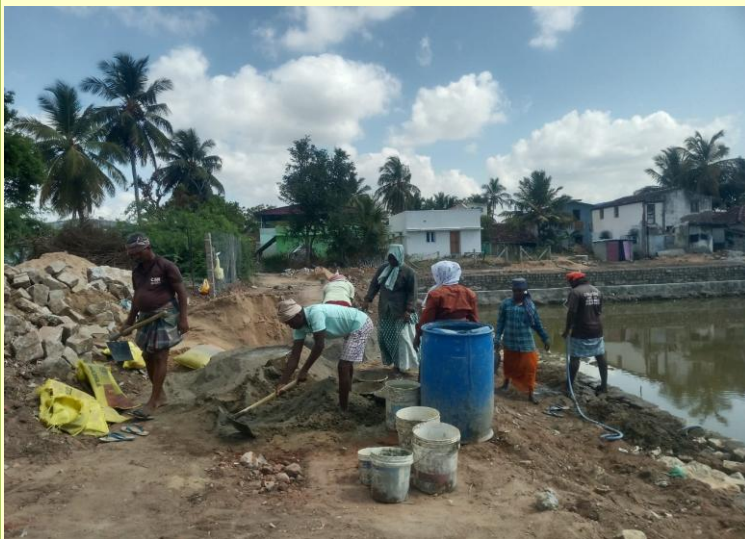
Workers at work for constructing the parapet wall
