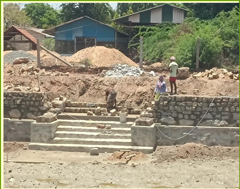
Construction of steps at the entry of the Teertham is on ..
