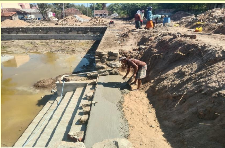
Mason giving finishing touches to the steps
