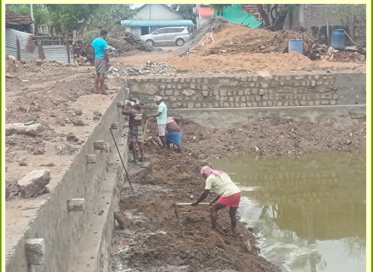
Strengthening and levelling work of the pond is on ..
