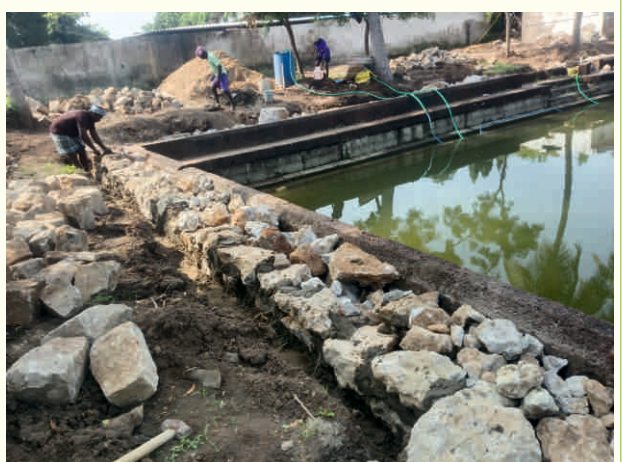
Construction of retaining wall is on .....
