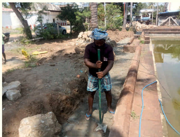
Preparing the ground for additional retaining wall
