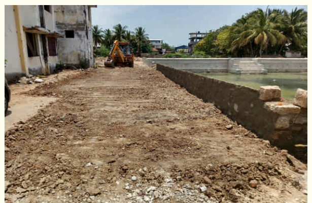
Levelling of Surrounding area
