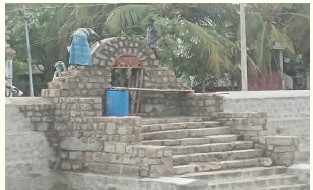
Entrance Arch construction
