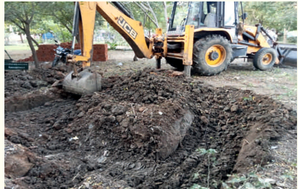
Earthwork for Foundation
