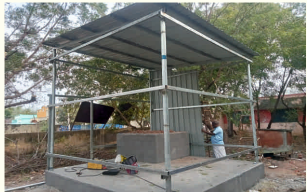
Shed construction is on
