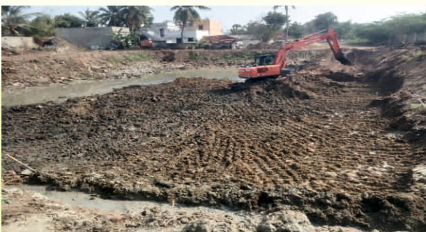
De-silting is on by using JCB
