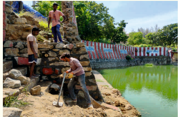
Stages of retaining wall construction
