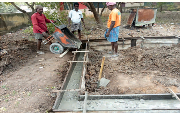
Foundation Concrete
