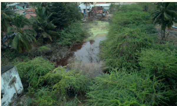
Condition of the Teertham
