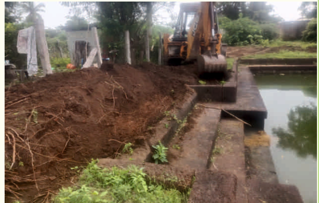
Cleaning the surrounding areas
