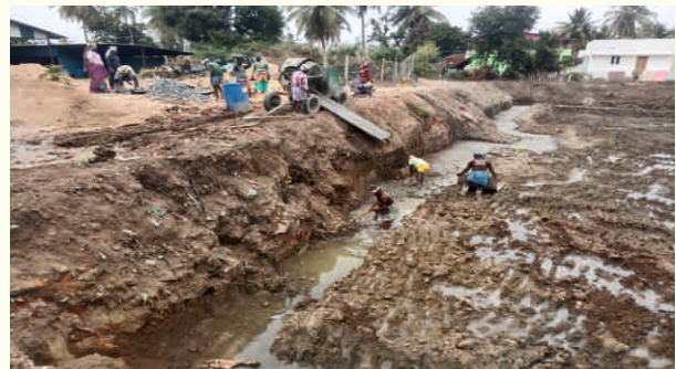
Foundation concrete work by chuting ( Ramp)
