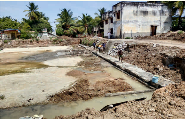
Retaining wall work is under progress
