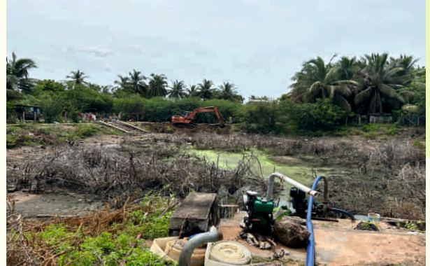
Cleaning of Thorny Trees & Draining the water
