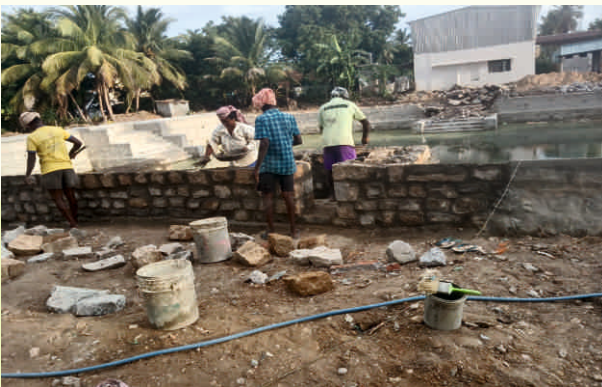
Parapet wall construction is on...
