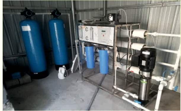
Installing R.O plant
