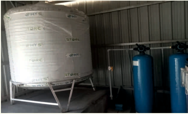
Installing R.O plant
