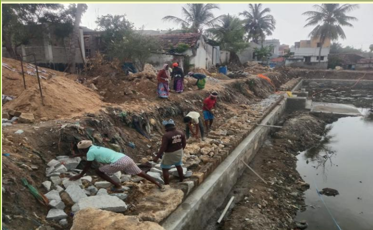
Strengthening the retaining wall is in the process ...
