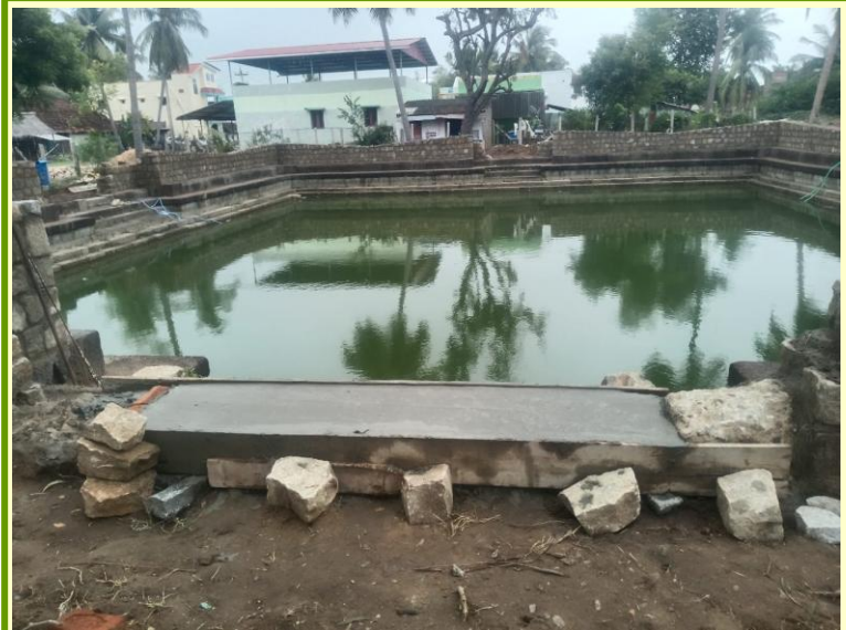
Creation of platform for constructing the Arch
