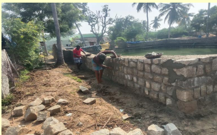
Pointing work of the side wall is on ...
