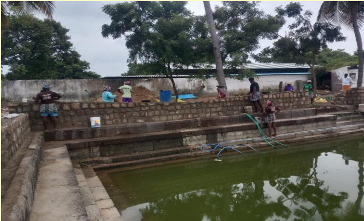
Workers are busy in constructing the Parapet wall
