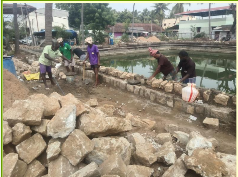
Recycling and Reusing the stones and boulders arranged from nearby areas for constructing the wall
