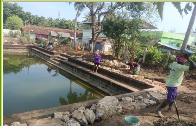
Masons are busy in arranging stones and boulders for erecting parapet wall
