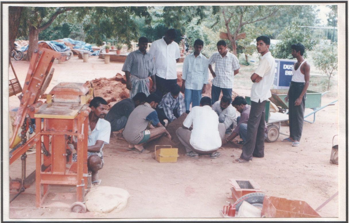
Mixing for Compressed Earth Block
