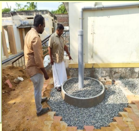
Shri. Ramakrishnan demonstrating "Rainwater harvesting structure" at site
