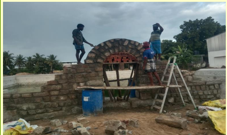
Entrance gate work is on ...
