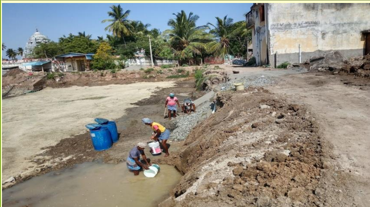
Removing the water and silt
