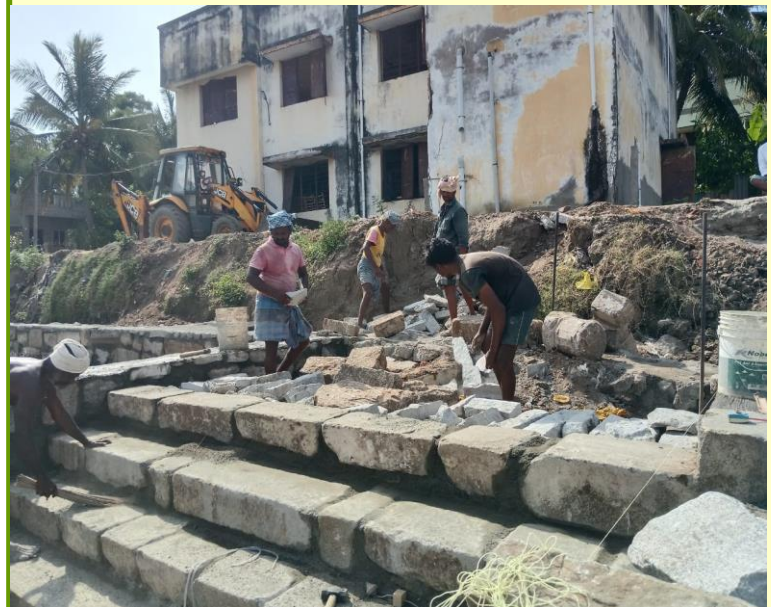
Construction of steps at the entry of the Teertham
