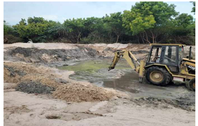
De - silting and Deepening the water body
