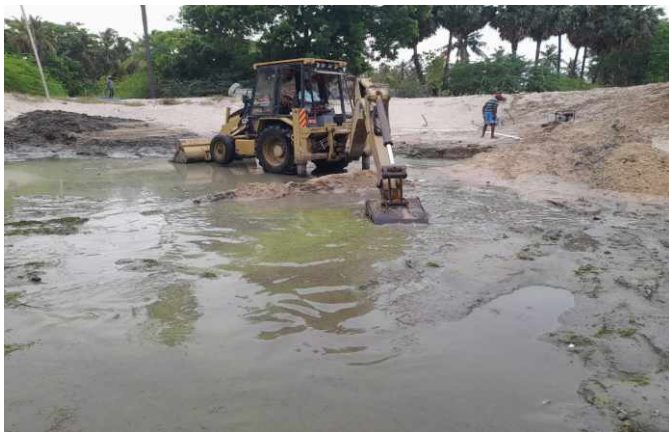
De - silting and Deepening the water body
