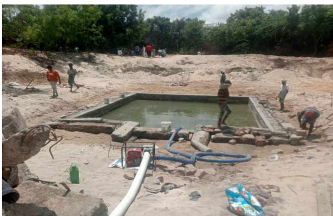
Construction of Inner pond and ring well
