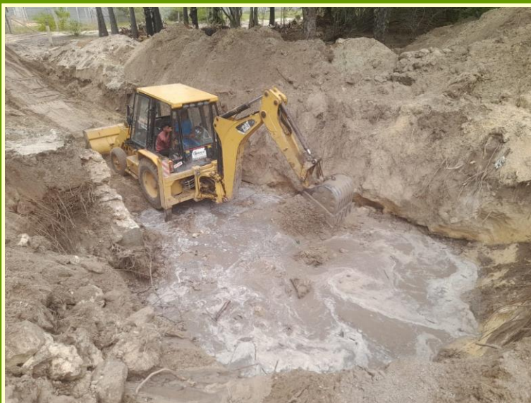
Removing the old sludge and deepening the water body
