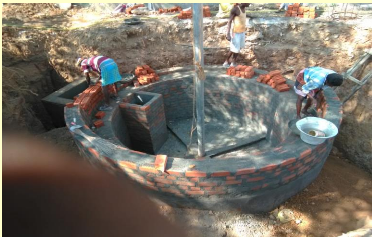
25 cum Shakti Surabhi Bio-methanation plant construction work is on at Ambattur, Chennai
