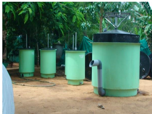
Different sizes of Shakti Surabhi Bio-methanation plants
