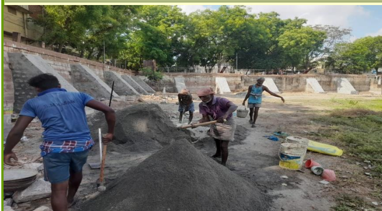
Workers are at work.. Background views of newly constructed piers for strengthening the walls
