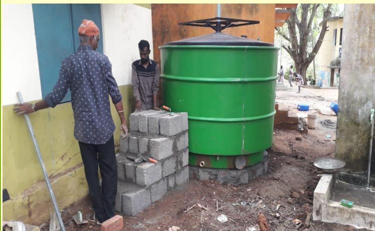
Finishing touches to the base and steps
