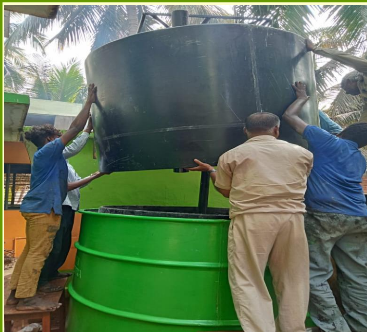
Fixing gasholder above the digester at Arunachala College, Kanyakumari district
