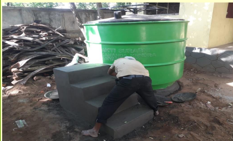
Step construction is on .. for easy pouring of input material to the Bio-methanation plant at Arumanallor
