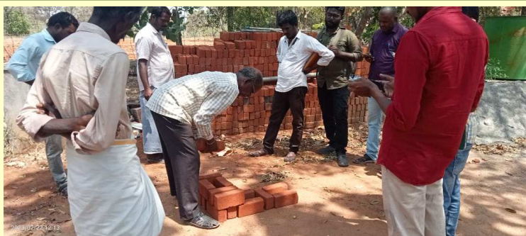
Shri.Muneeswaran demonstrating Rat trap model construction
