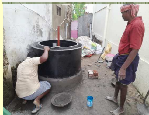
Unloading of Shakti Surabhi digester and gas holder
