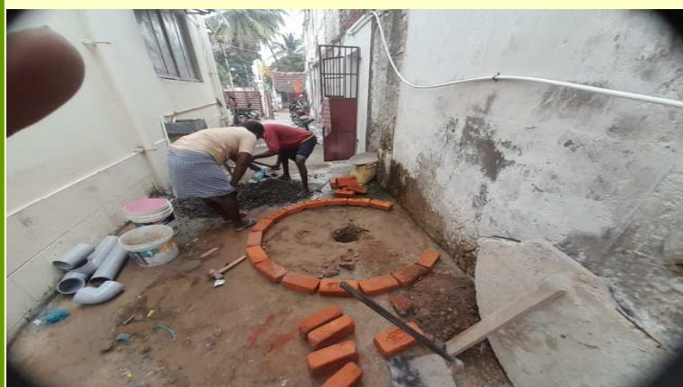
Preparation of platform for installing Bio-methanation plant
