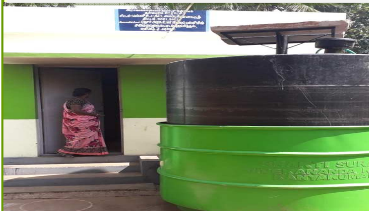
Commissioned plant with full of gas with dead weight on the top to get pressure at the biogas stove -Govt. High school, Pudhur
