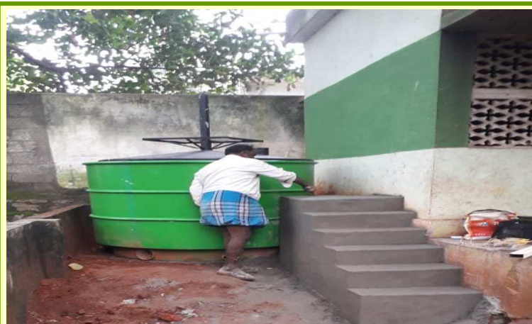
Masons preparing steps for easy pouring of input materials at Govt. High school, Peyankuzhi, Kanyakumari Dist.
