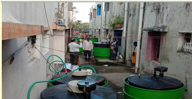
Installation of Biogas plants in the crowded lane - a typical urban scene
