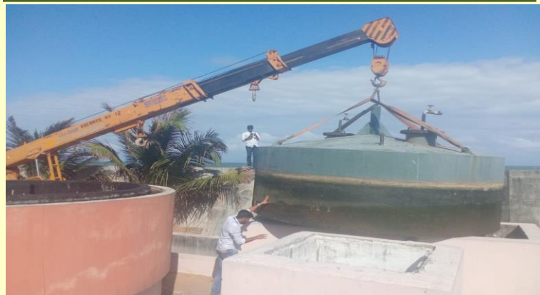
Lifting of gasholder with the help of crane for maintenance
