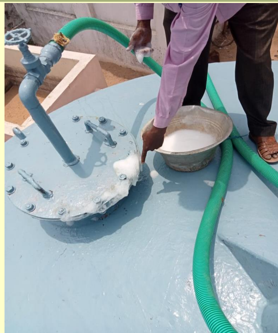
Checking of gasholder and pipeline with traditional method of using soap water
