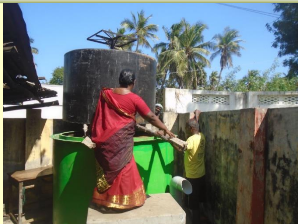
Commissioning of Bio-methanation plant - feeding the slurry and then installing the gas holder above the digester
