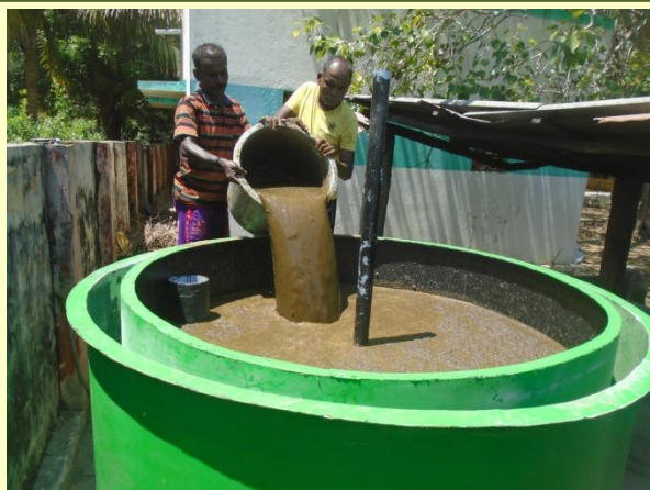
Commissioning of Bio-methanation plant - feeding the slurry and then installing the gas holder above the digester
