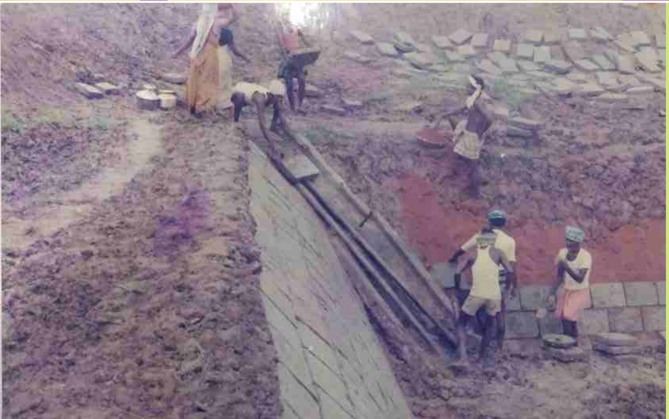
A novel method of pitching the slopes with stones to avoid sliding of the soil
