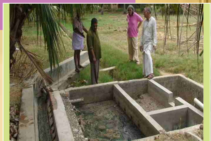
Sedimentation and Filtration tank
