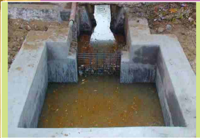
Sedimentation and Filtration tank
