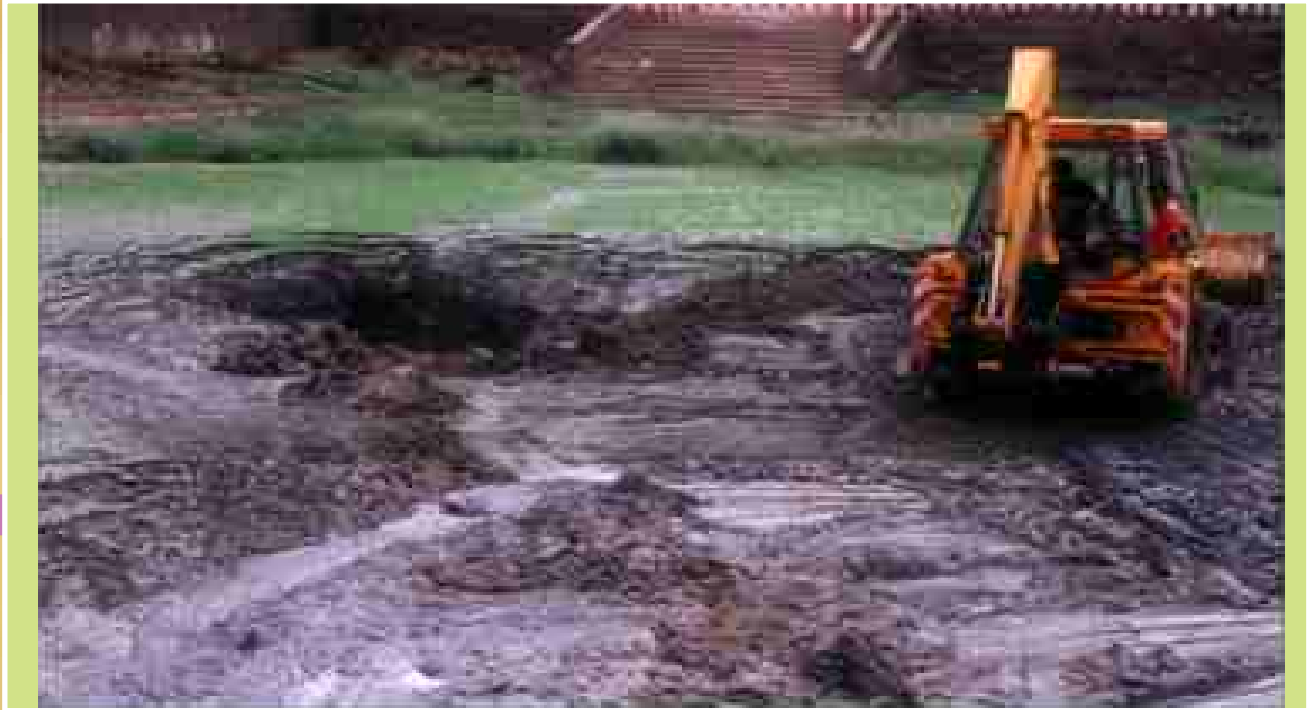
JCB is clearing the silt accumulated over the years
