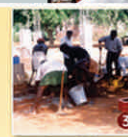
Dry mixing sand, soil & cement
