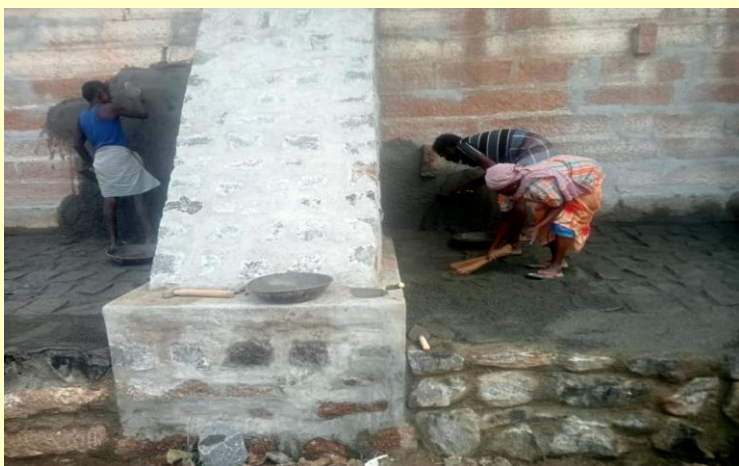
Strengthening the wall by piers and additional support by joining the piers
