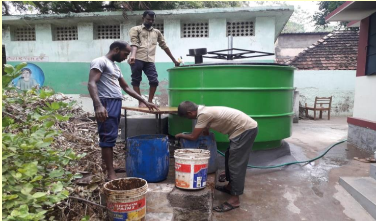
Mixing cow dung into slurry before pouring to the Bio-methanation plant at Govt. Middle school, Parakkai
