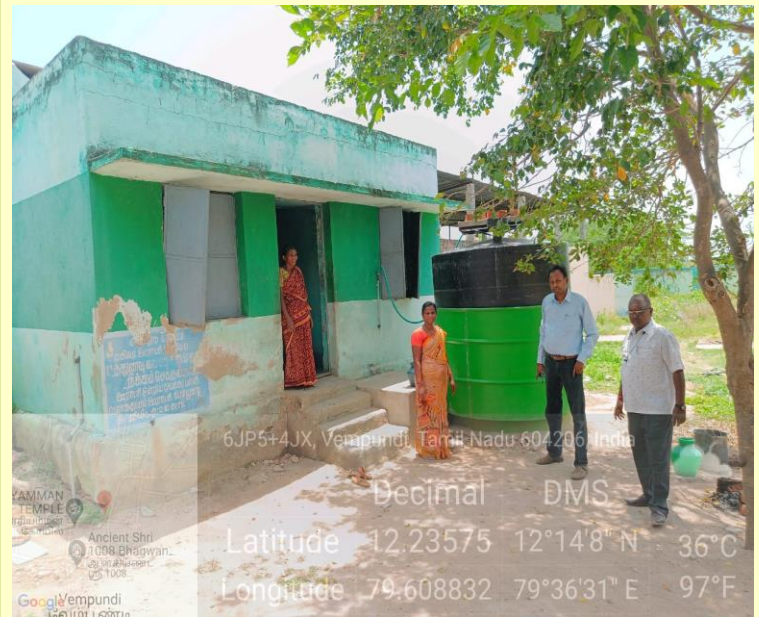
Assistant Executive Engineer, Dindivanam inspected the working of Bio-methanation plant at Vempundi school at Pelakuppam Panchayat, Villupuram district
