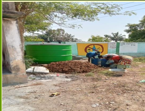
Preparing cow dung slurry with devotion for commissioning the plant at Government High school, Agoor, Villupuram Dist.
