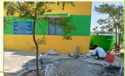
Plumbing work is on at Government High School, Devanur, Villupuram Dist.
