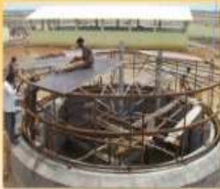
Gas Holder work is on
